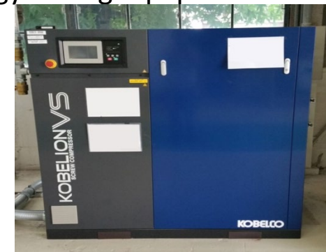
Upgraded to the latest compressor(w/ highly efficient , visualization system)
