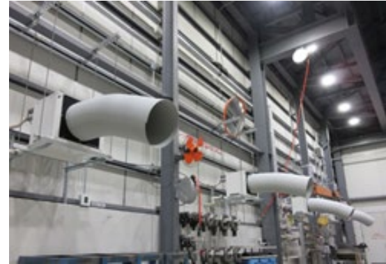
eg. Higher-efficient air conditioning (individually controllable, ductless multi-
