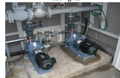
Top runner spec.(best energy efficient) pump unit 8
